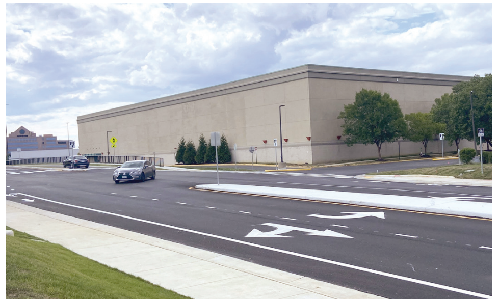
Part of the new section of Government Center Parkway, with a raised median, turning lanes, bike lanes and crosswalks.
